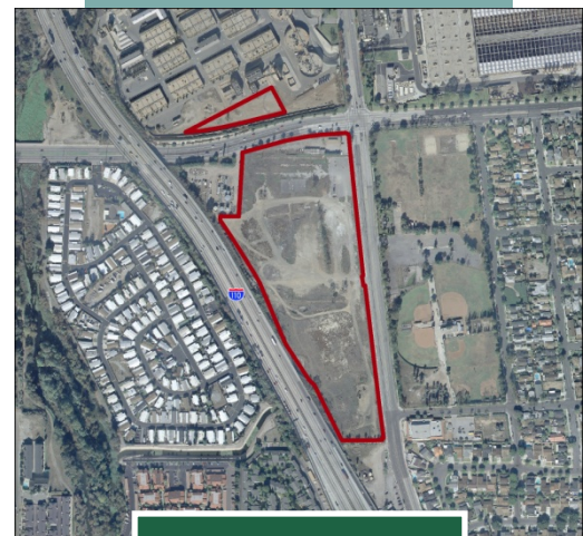
JWPCP West Shaft Site
