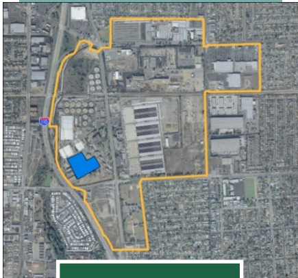
Joint Water Pollution Control Plant
