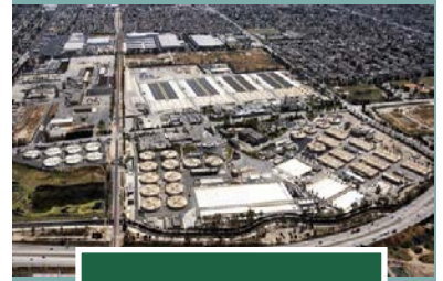
Joint Water Pollution Control Plant
